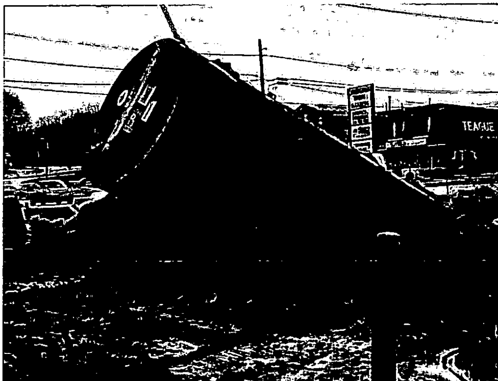
PHOTOGRAPH 2. View showing the removal of the 8,000-gallon tank.
