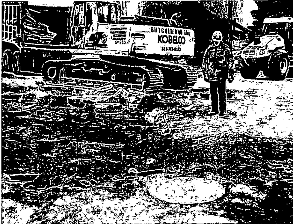
PHOTOGRAPH 3. View showing the coverplate for the water well. Concrete removed from the dispenser island area just north of the UST excavation. Photo is facing south.
